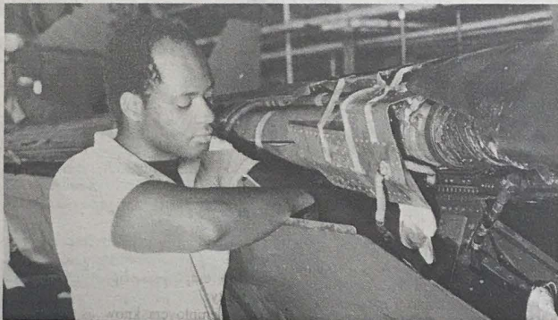
SSgt. Rodney A. Hall reconnects the flap actuator switch on an engine. An aircraft electrician, Sergeant Hall is performing a phase inspection procedure, after a beef-up plate was installed on the wing flap. The switch tells whether the flap is up, down or in transit.
